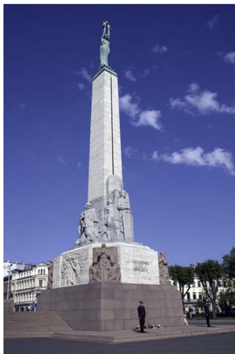
Figure 28. Freedom monument, Riga (Lettonia) Restored using polyurethane resins mainly, for sealing purposes. [39] (by courtesy of Latvian Tourism Development Agency).
