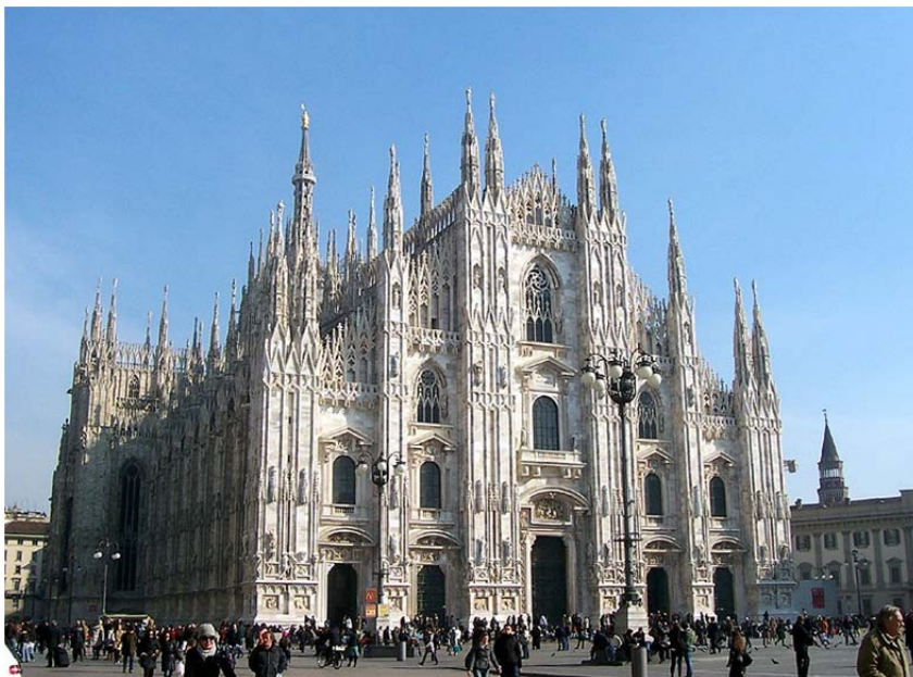
Figure 25. Milano dome (Italy) Restored in 1972 using epoxy resins mainly, for sealing purposes, together with acrylic resins [32] (By courtesy of MarcusMark http://it.wikipedia.org/wiki/File:876_MilanoDuomo.JPG (03.06.2013)).
