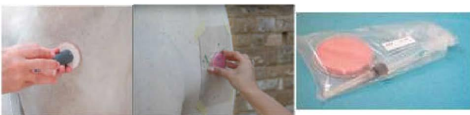
Figure 3. Some examples of “in situ” contact sponge measures and the kit available from CTS, Altavilla Vicentina (Italy).
