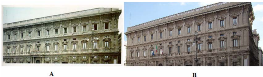
Figure 20. Marino Palace, Milan. Ceppo Gentile sandstone before restoration (A) and after restoration with Rhodorsil RC70 and Silirain 50 (1989), two polysiloxanes (B). (By courtesy of Friedrichstrasse http://it.wikipedia.org/wiki/File:Milano_pal_Marino_piazza_Scala.jpg (03.06.2013)).
