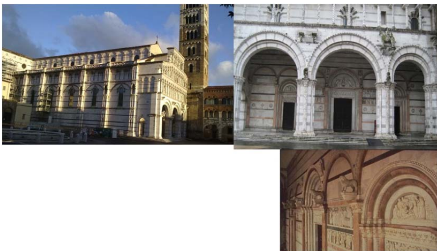
Figure 31. The Cathedral of St Martin ( Duomo di Lucca ) and its bell tower in Lucca, Tuscany, Italy, S Giuliano Marble, red nodular ammonitic limestone from Alta Garfagnana, deep green serpentine from Prato, restored with Fomblin Met (1982). [42f] (by courtesy of Diocesi Lucca- Italy)
