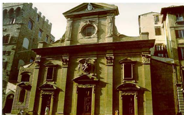
Figure 35. St Trinita Church, Florence. Pietra Forte restored with IBA and a fluoroelastomer (1990-92).
