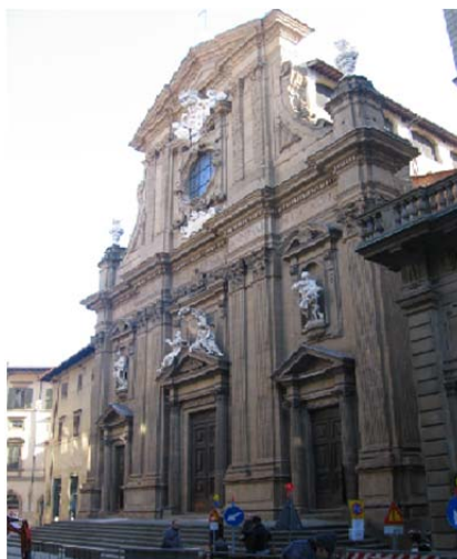
Figure 36. St. Michele and Gaetano Church, Florence. Pietra Forte restored using an acrylsiliconic resin, Akeogard CO and Akeogard BA (1991-96). [43]
