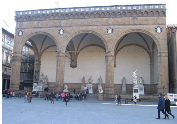
Figure 34. Loggia dei Lanzi, Florence. Protected using Akeogard BA, ceilings with Akeogard CO (1988 -90).
