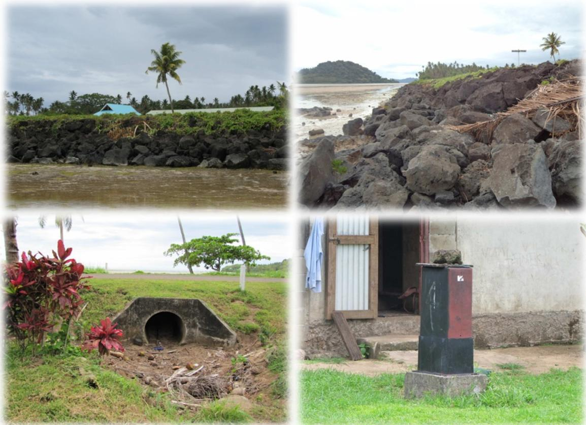
*Photos of Naselesele Village, showing the seawall (top), culvert across the main coastal road (lower left) and elevated power junction box (lower right)*
