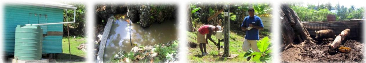
Yanuca Village water sources (L-R): rain catchment; groundwater catchment; borehole; pig sty above catchment
