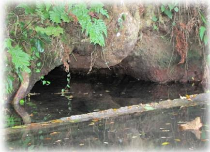
Naselesele village also has a spring source for water that has been used by past generations. This spring is well maintained with a cement wall water collection and protection. During high tide this spring is flushed with minimal seawater and is used for bathing, washing and drinking. The water resources for Naselesele are summarized in Figure 2.
