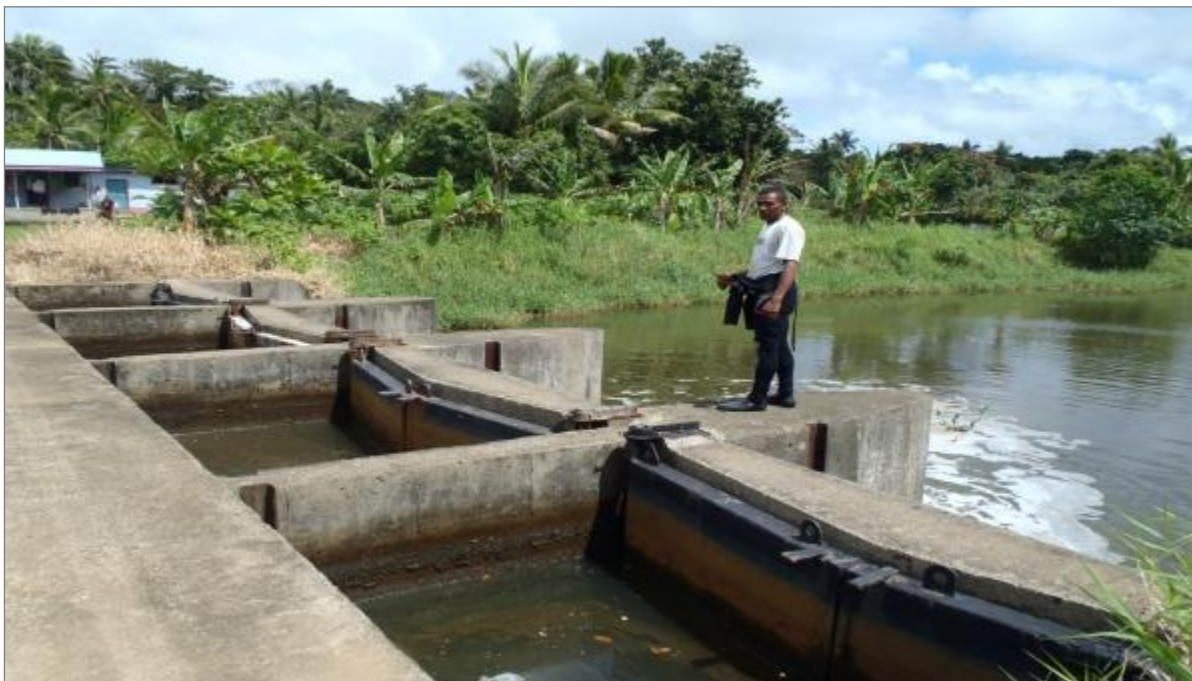
Figure 27: Floodgate in the Waicoka river system
