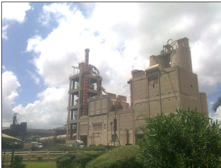
Figure 1. Cement production plant (Cement company, Zimbabwe).
