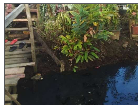
Figure 4: Stagnant water guttering
