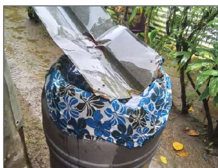
Figure 3: Rainwater collection and guttering
