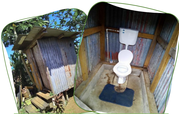
Examples of the toilets surveyed in Namadi
