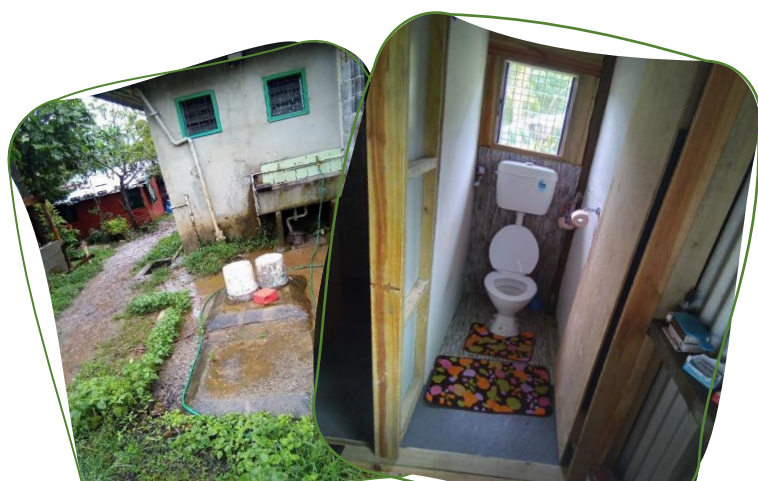
Examples of the toilets surveyed in Ragg Avenue
