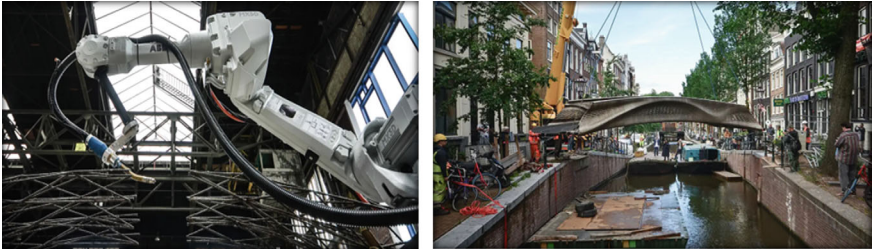
Fig. 5 RA3DP printed bridge (Block 2018)
