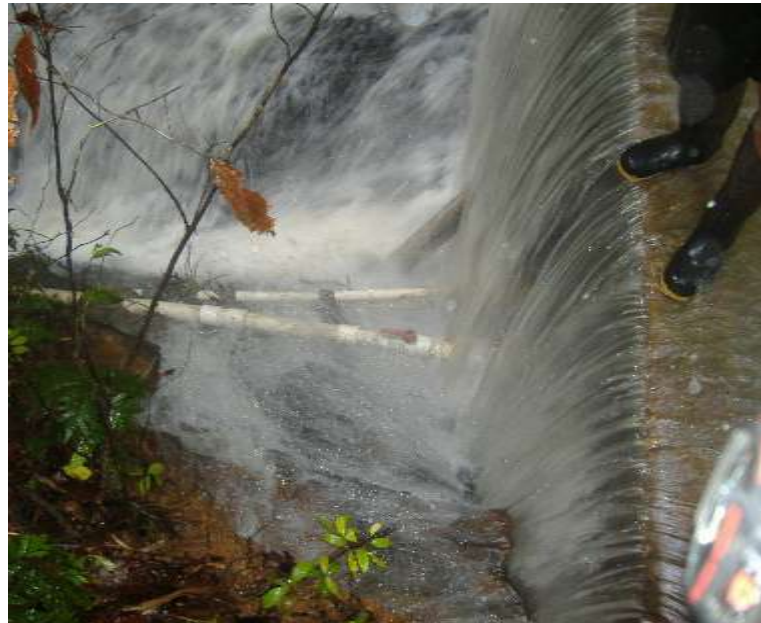
Nanohydro dam at Tiko's farm, Savu village, Fiji
