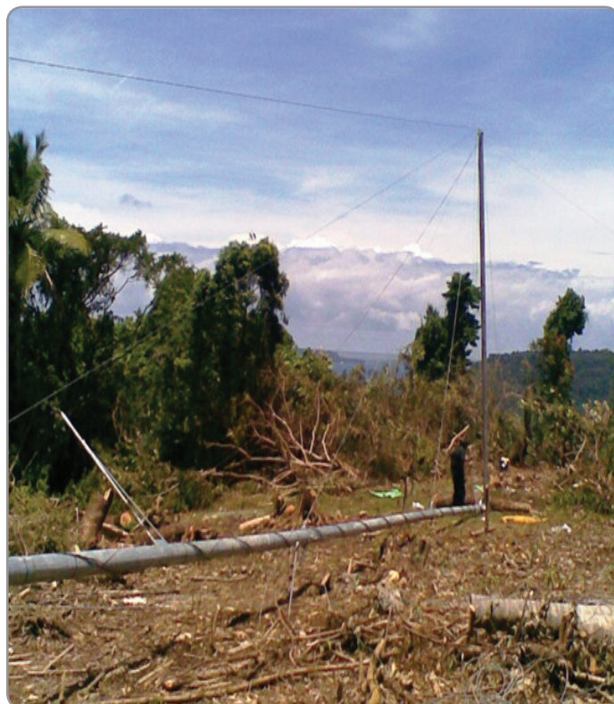
Figure 12: Wind monitoring mast installation in Port Olry
