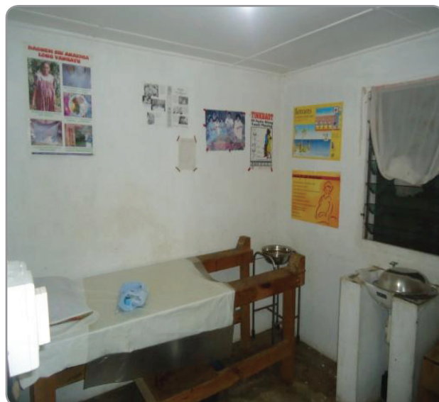
Figure 8: PV system at Tasmulum Dispensary
