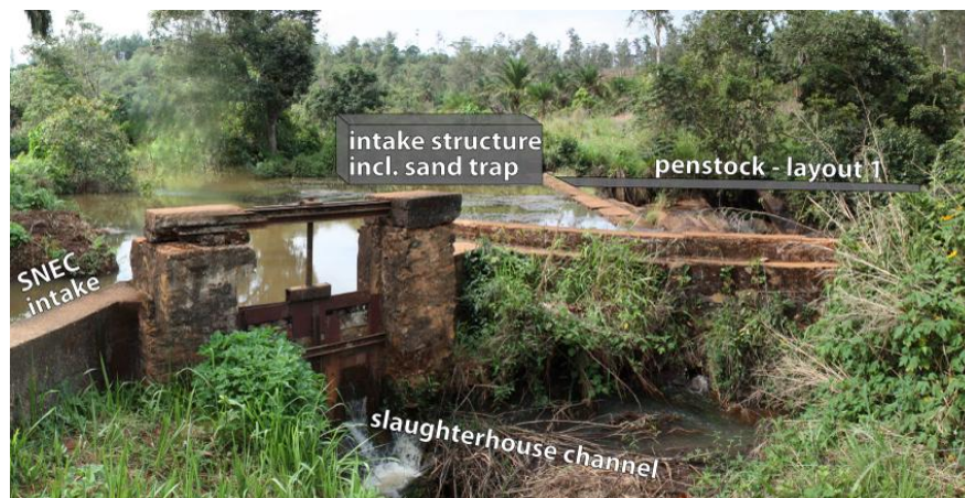
Fig. 15 Overview of intake situation at “cascade_1”
