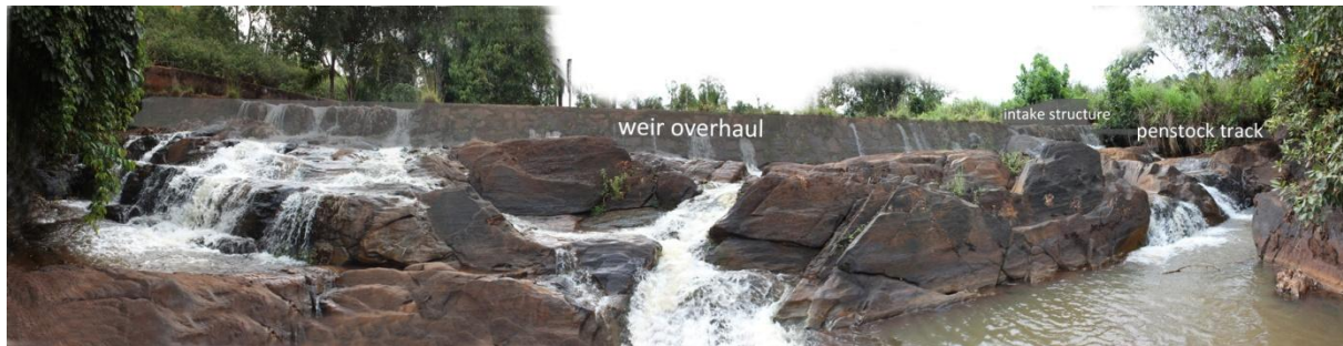
Fig. 7 Downstream view with weir overhaul and intake structure
