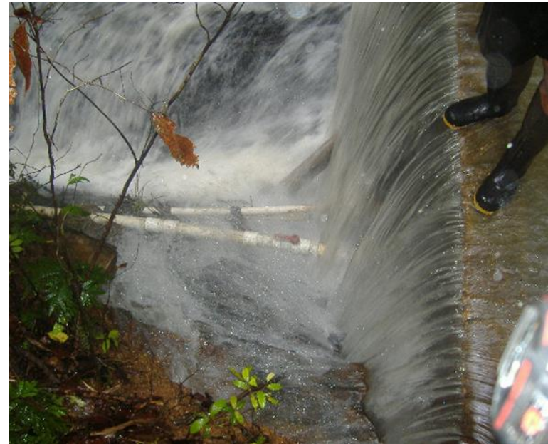
A 44W nano-hydro scheme at Tiko's farm, Savu village, Fiji
