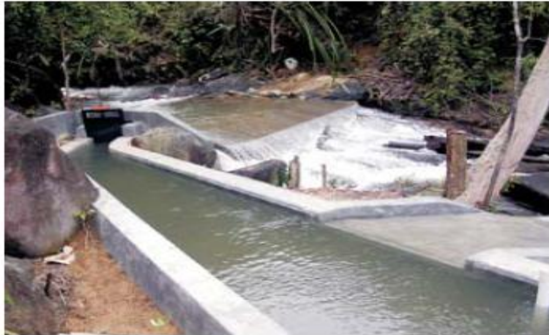
Photo 2. Intake structure of the Sadap MHP rural electrification scheme financed through district government development funds.
