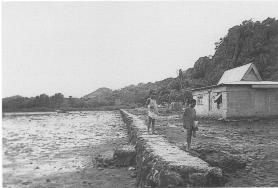
Figure 3. The shoreline at Nasauvuki Village, Moturiki Island, Fiji. Problems of shore erosion and flooding have been caused largely by mangrove clearance. Mangroves are growing back but are pulled out when they get about 0.5m in height. The seawall is typical. The house has a raised front door, but water still spills over the doorstep at high tide. Tidal range is about one meter. This site faces a reef-enclosed lagoon.
