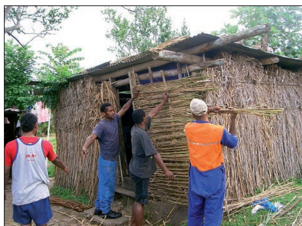
Figure 2. Local house being renovated in Dravo.
