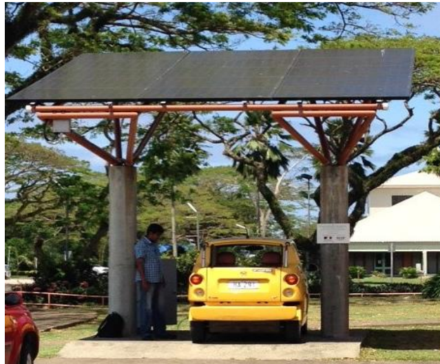
Figure 3. The solar charging station roof mounted panels with two supports to allow for vehicle parking and charging area
