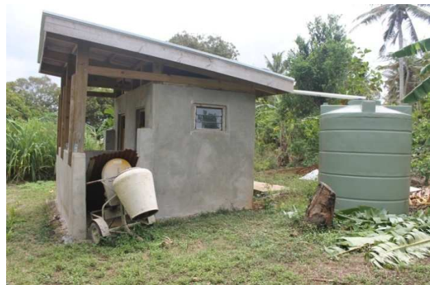
Photo: Community toilet facility
